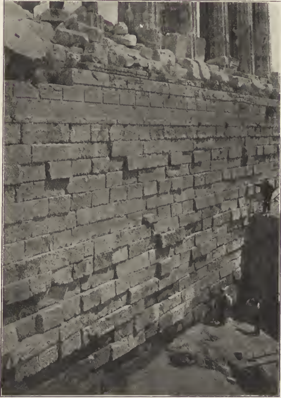
FIG. 32.—Courses of the Foundation Walls of the Parthenon, south side.
